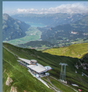
Alpen tower Hasliberg
